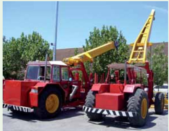
Onsite cranes assist in the unloading of raw materials.
